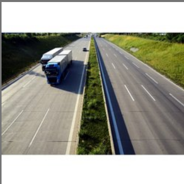
Airtel Vehicle Tracking Solution
